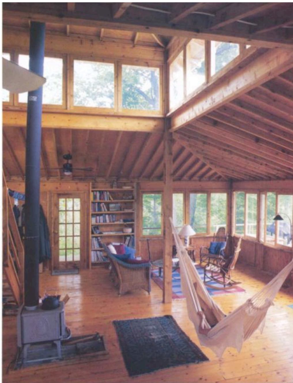
A seasonal cottage means simplified details. With no insulation in the walls or ceiling, the inside of the sheathing and the exposed framing lend a rustic feel to the cottage's light, open interior. Photo taken at A on floor plan.
