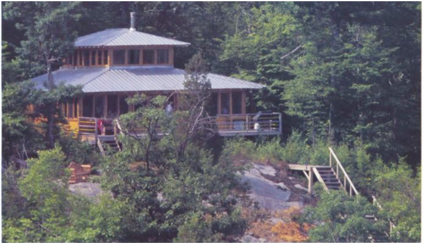
A steep climb from the driveway to the front door. Added after the house was completed, a long staircase makes the climb up the granite face easier. The builders didn't have that advantage when they were hauling materials to the top of the hill. Photo taken at B on floor plan.
